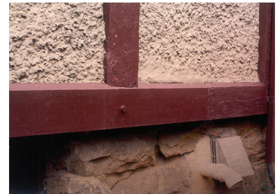
Below: Close up photo of the new stucco and band board, applied with care, to restore the original appearance of the wall.
