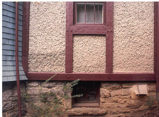
Below: The inappropriate repairs were removed. Stucco which matches the original was applied and a band board milled and beveled to match the existing was installed.
