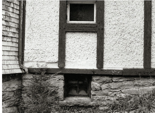
Above: Deteriorated pebbledash/roughcast stucco and a rotten band board were replaced by inappropriate materials - smooth plaster and an undersized board.
