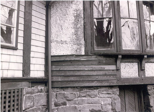
Above: Instead of repairing deteriorated stucco with fresh pebbledash/roughcast stucco, wood lap siding was used.
