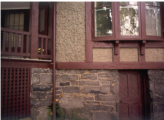
Below: The lap siding was removed and the half-timbering and stucco were repaired to restore the original appearance.
